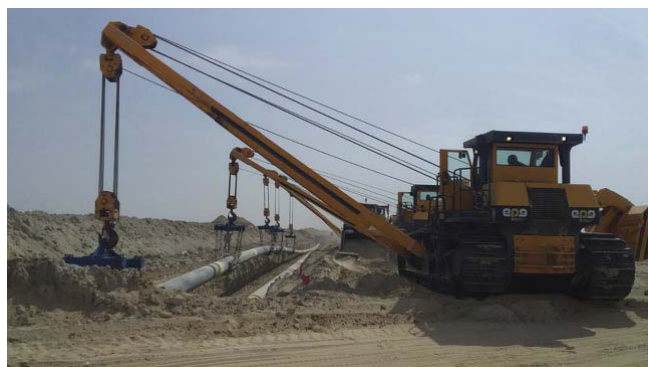
Figure 1. Performer 980 laying pipe in Kuwait.
