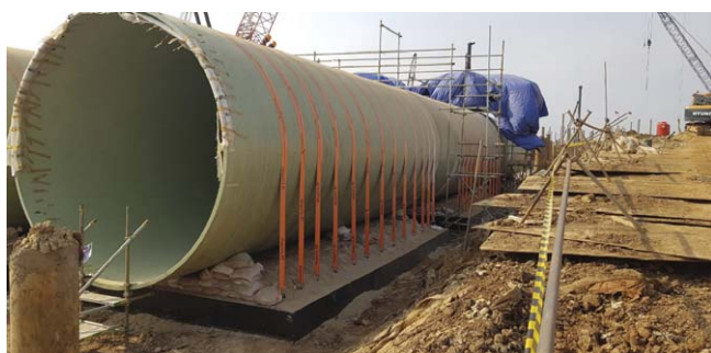
Figure 7. Platipus system to prevent uplift used in combination with foundation on the Cirebon 2 project, Indonesia.
