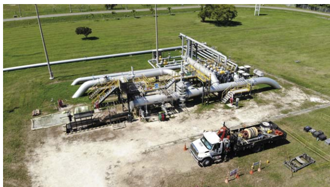
Figure 2. Loading lines only have one launch-receive site, which makes BIDI ILI necessary.
