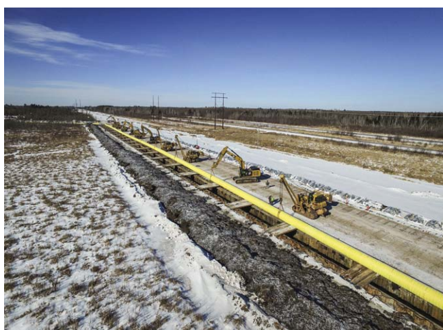
Figure 2. Crews worked 24 hours a day to install sheet piling and welding/stringing the replacement section in sub-zero temperatures.
