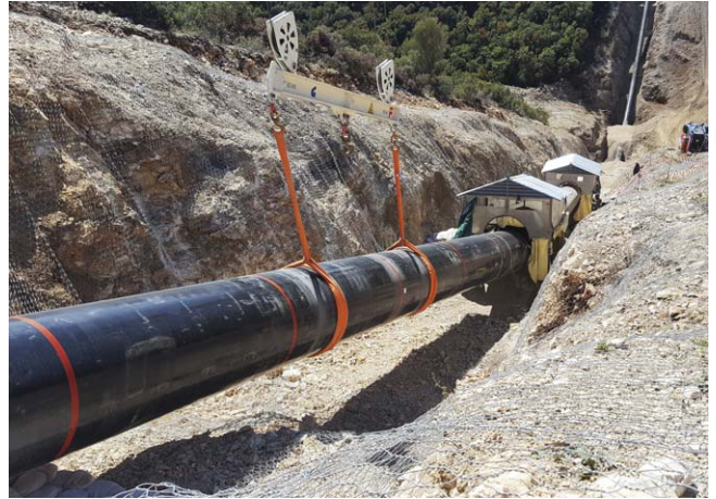
Figure 4. Precise positioning of the pipe for welding purposes.
