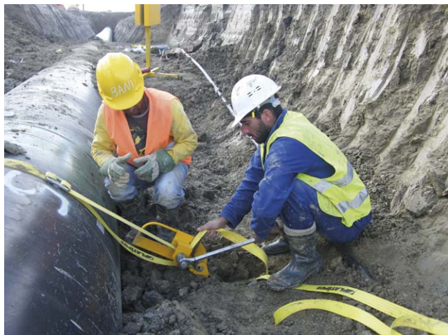
Figure 5. Platipus pipeline anchor system being tensioned on the TAP project in Albania.
