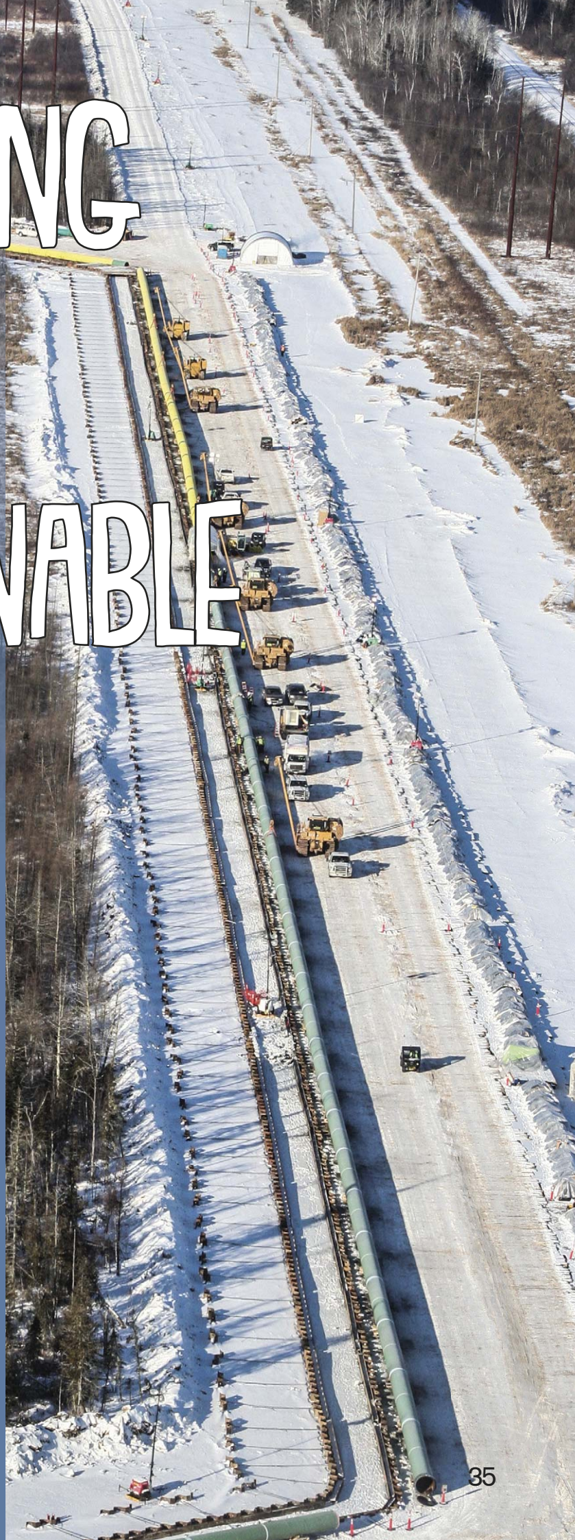
Figure 1. A 2.25 mile ice road through an expansive wetland was maintained at 24 - 40 in. of frost and ice.
