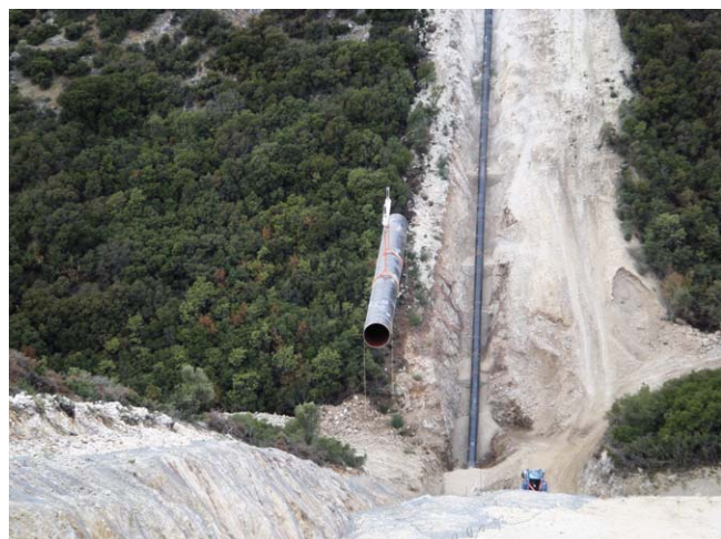
Figure 2. Transport of 48 in. pipes in up to 30° inclined terrain for a pipeline project in Greece.
