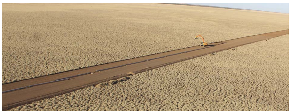
Figure 6. Unloading and stringing pipeline near Mount Isa.
