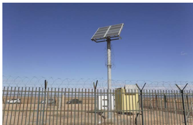
Figure 1. One of the ICCP stations on the Hassi R'Mel pipeline in Algeria.
