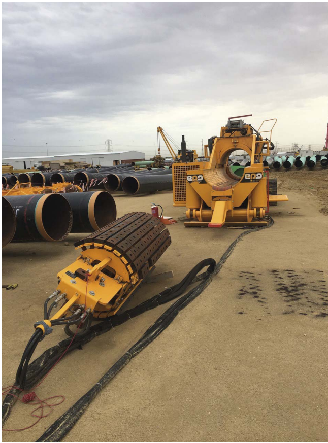
Figure 3. Euro Pipeline's 22-36 bending machine and mandrel ready for bending.
