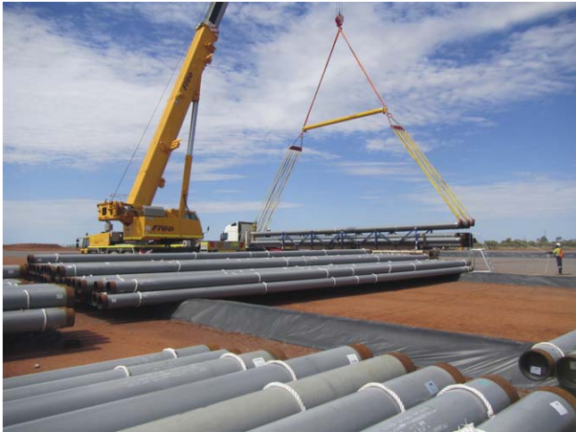
Figure 2. More than 33 000 lengths of pipe were used to construct the Northern Gas Pipeline.
