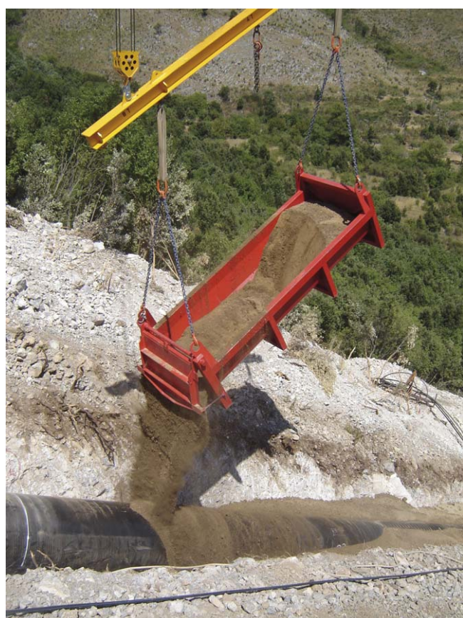
Figure 3. Easy transportation of padding material for filling up the trenches. Due to the two independent lifting systems of the crane unit the bulk can be adjusted as required.
