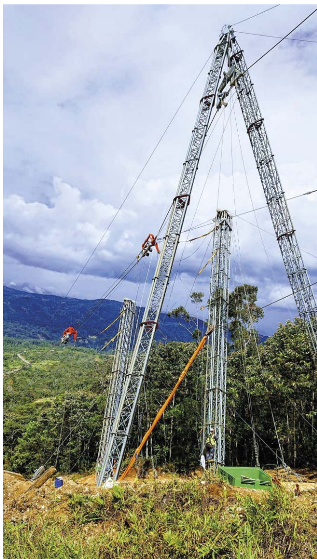
Figure 7. Case study in Papua New Guinea, where two cable crane systems are installed on different steep slope sections.
