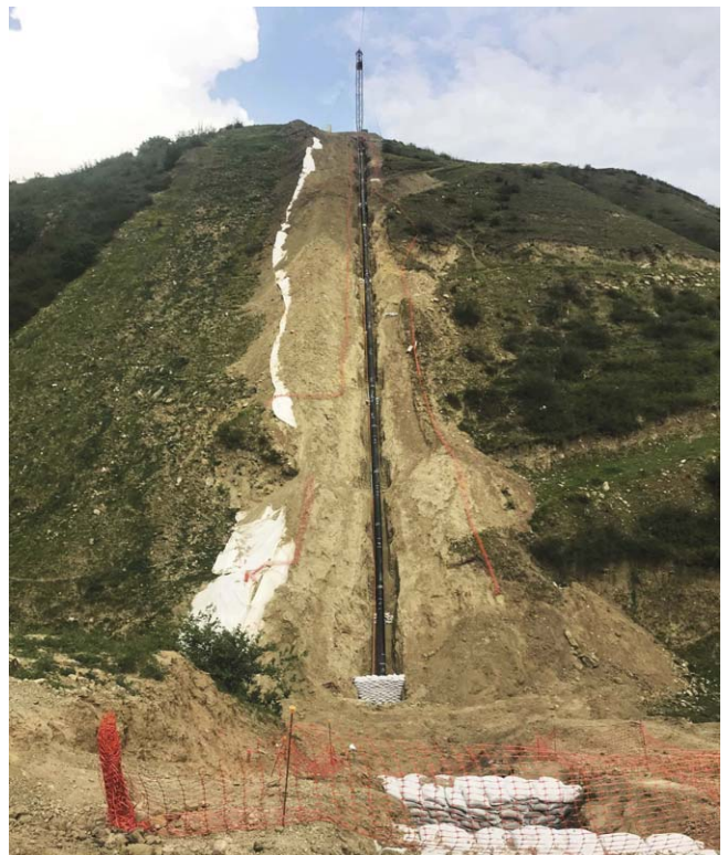
Figure 5. Cable crane systems require a smaller ROW than traditional methods, which means the environmental impact is reduced.
