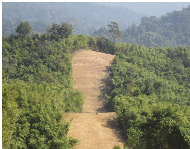
Figure 6. A reinstated steep slope by means of a cable crane system and spider excavators after the pipeline construction has been finished.
